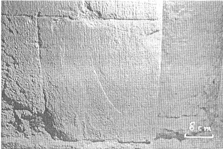
Fig. 1: Sandstone of Kordel: granular disintegration
