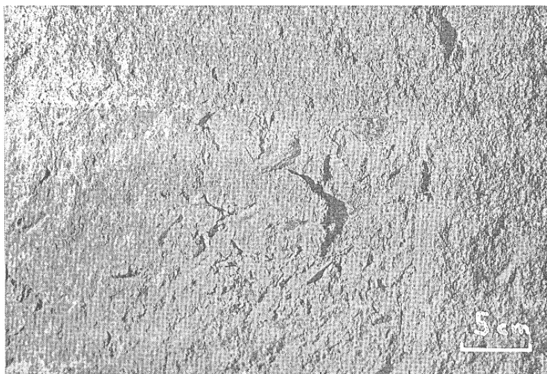
Fig.3: Drachenfels Trachyte: scaling in fragments up to hand-size
