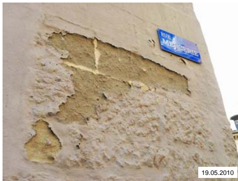
Materials and conservation of built cultural heritage – The weathering of the natural building stones. BR 64
