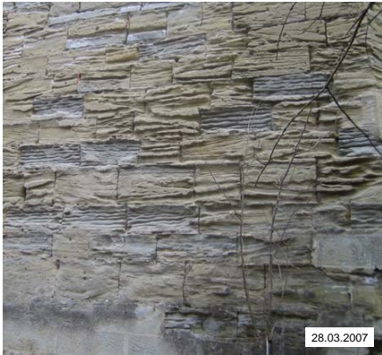
Materials and conservation of built cultural heritage – The weathering of the natural building stones. BR 07
