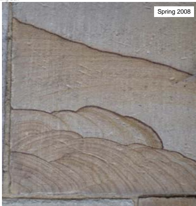
Materials and conservation of built cultural heritage – The weathering of the natural building stones. BR 2/9
