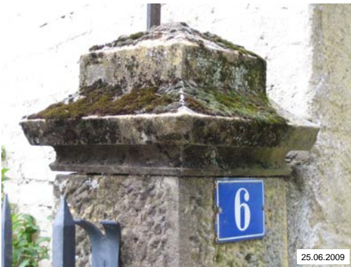
Materials and conservation of built cultural heritage – The weathering of the natural building stone. BR 89
