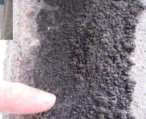
Stone materials and conservation of the built heritage - The soluble salts - BR /19
