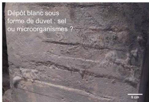
Stone materials and conservation of the built heritage - The soluble salts - BR /13
