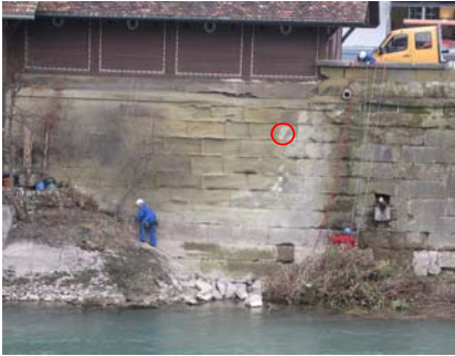
Degradation of Bernese sandstone by salts from concrete
