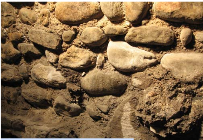
Boulder masonry, around 450 AD, St. Stephan, Chur, GR
