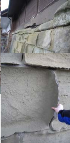
Degradation of Bernese sandstone by salts from concrete
