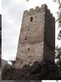
Materials and conservation of built cultural heritage – module 03
