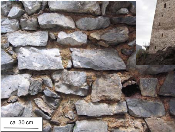
Meiringen, BE, Resti, 14.10.08, Rough stone masonry
