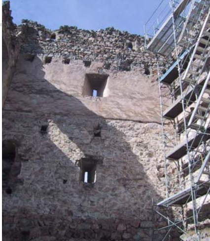
Materials and conservation of built cultural heritage – module 7/3
