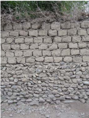
Mixed pebble and mud and mud brick wall
