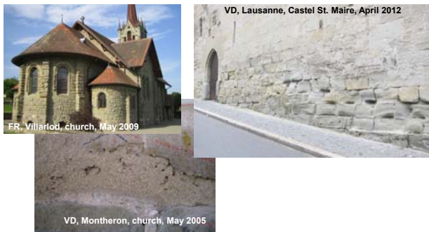
Stony materials and conservation of the built heritage – Petrology – BR 41
