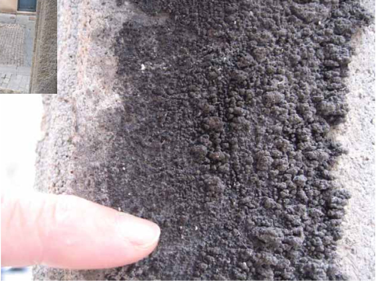
Nancy, 7.6.2008 Black crust of gypsum on the Euville limestone
