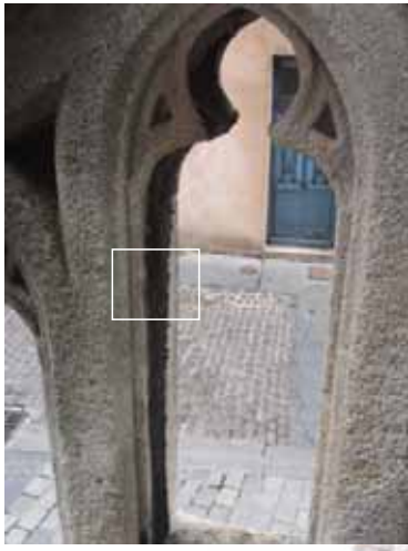
Nancy, 7.6.2008 Black crust of gypsum on the Euville limestone
